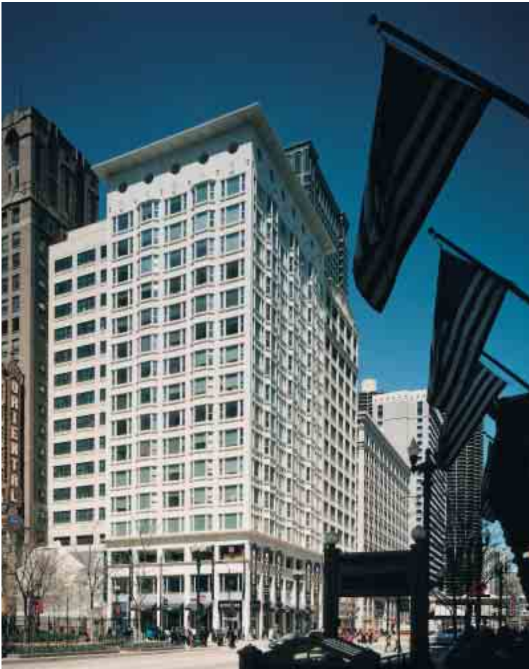
Located in downtown Chicago, the new residence hall for the School of the Art Institute is clad in GFRC panels, which emulate the look of the Windy City's historic buildings finished in terra cotta. The dormitory is composed of two connected buildings and a rear link. Photo: ©Brian Fritz Photography
